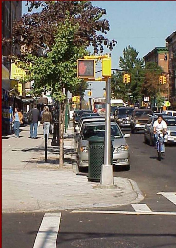
Parking aligns with curb extension, giving pedestrians a view of oncoming traffic
